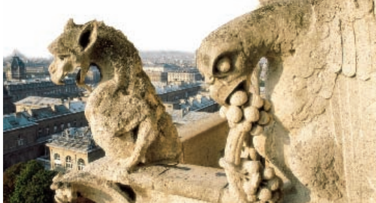
FIGURE 4 Effects of Chemical Weathering Acid rain chemically weathered these stone gargoyles on the cathedral of Notre Dame in Paris, France.
